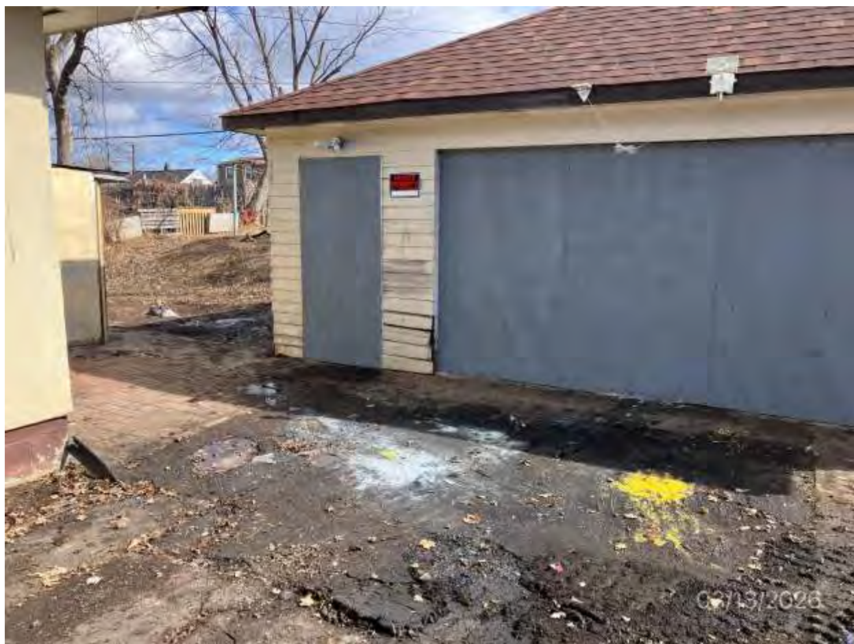
1164-1166 Cumberland St. Photos Before/After Clean Up 3-30-26
