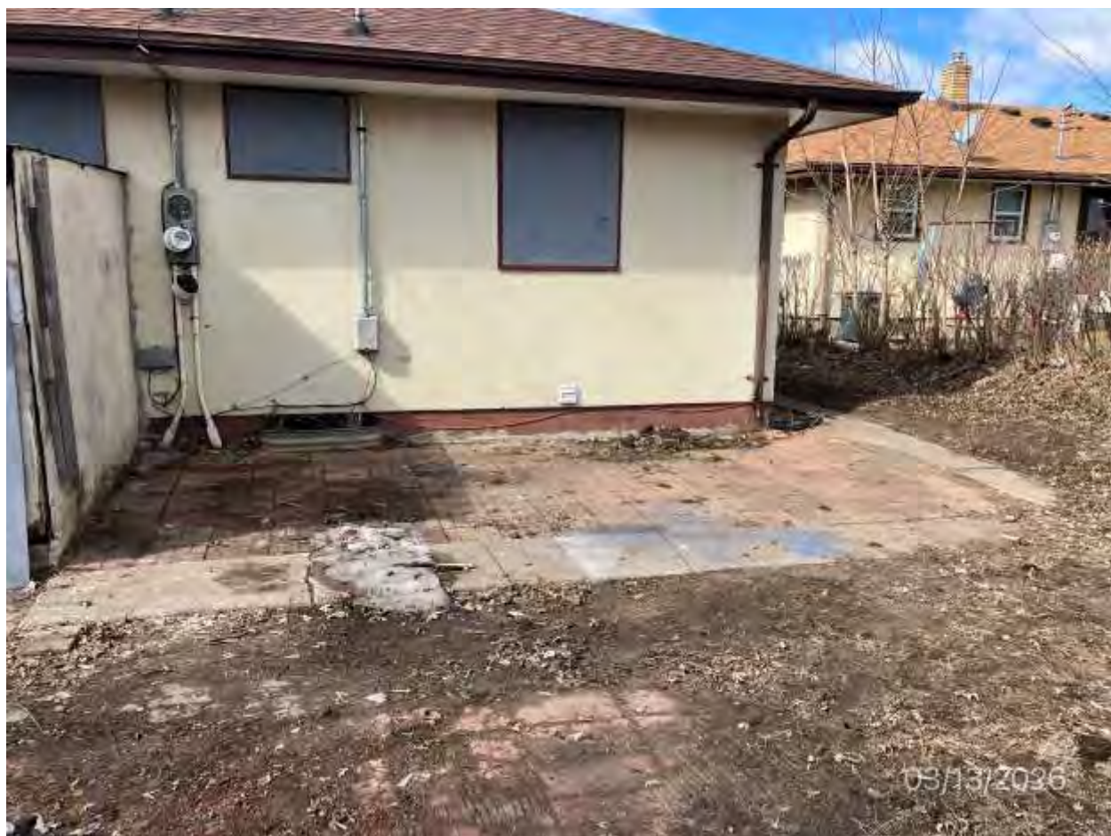
1164-1166 Cumberland St. Photos Before/After Clean Up 3-30-26
