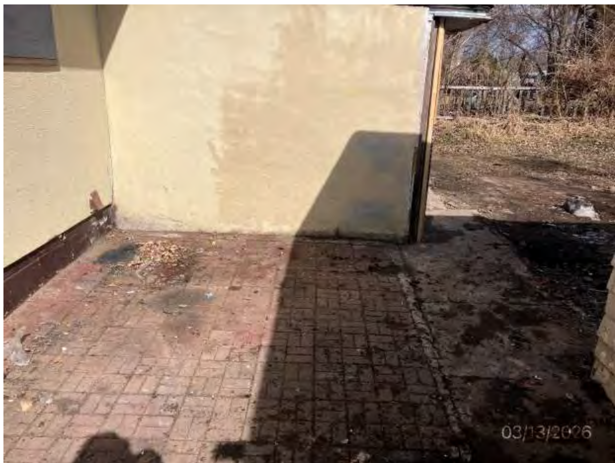
1164-1166 Cumberland St. Photos Before/After Clean Up 3-30-26
