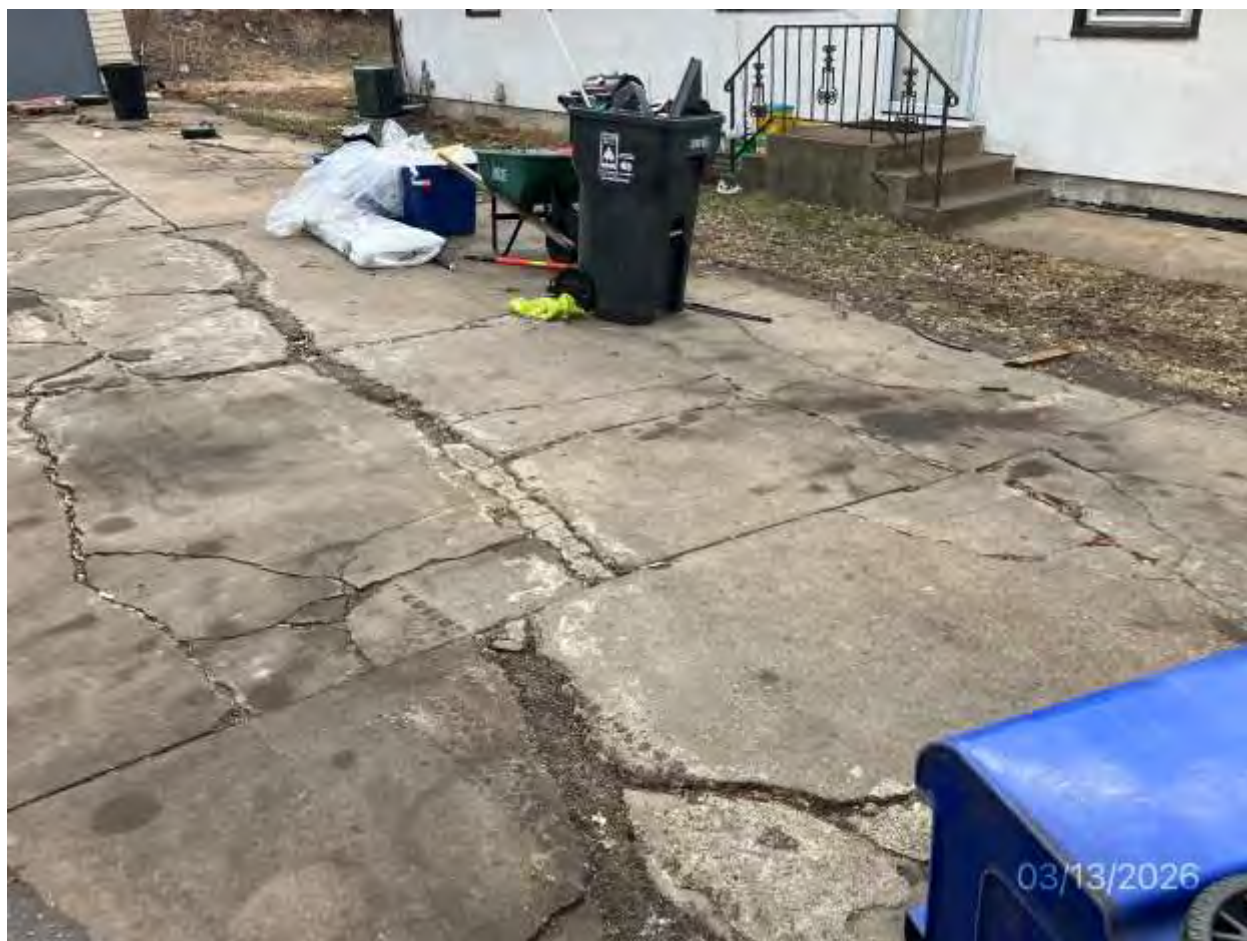
1164-1166 Cumberland St. Photos Before/After Clean Up 3-30-26
