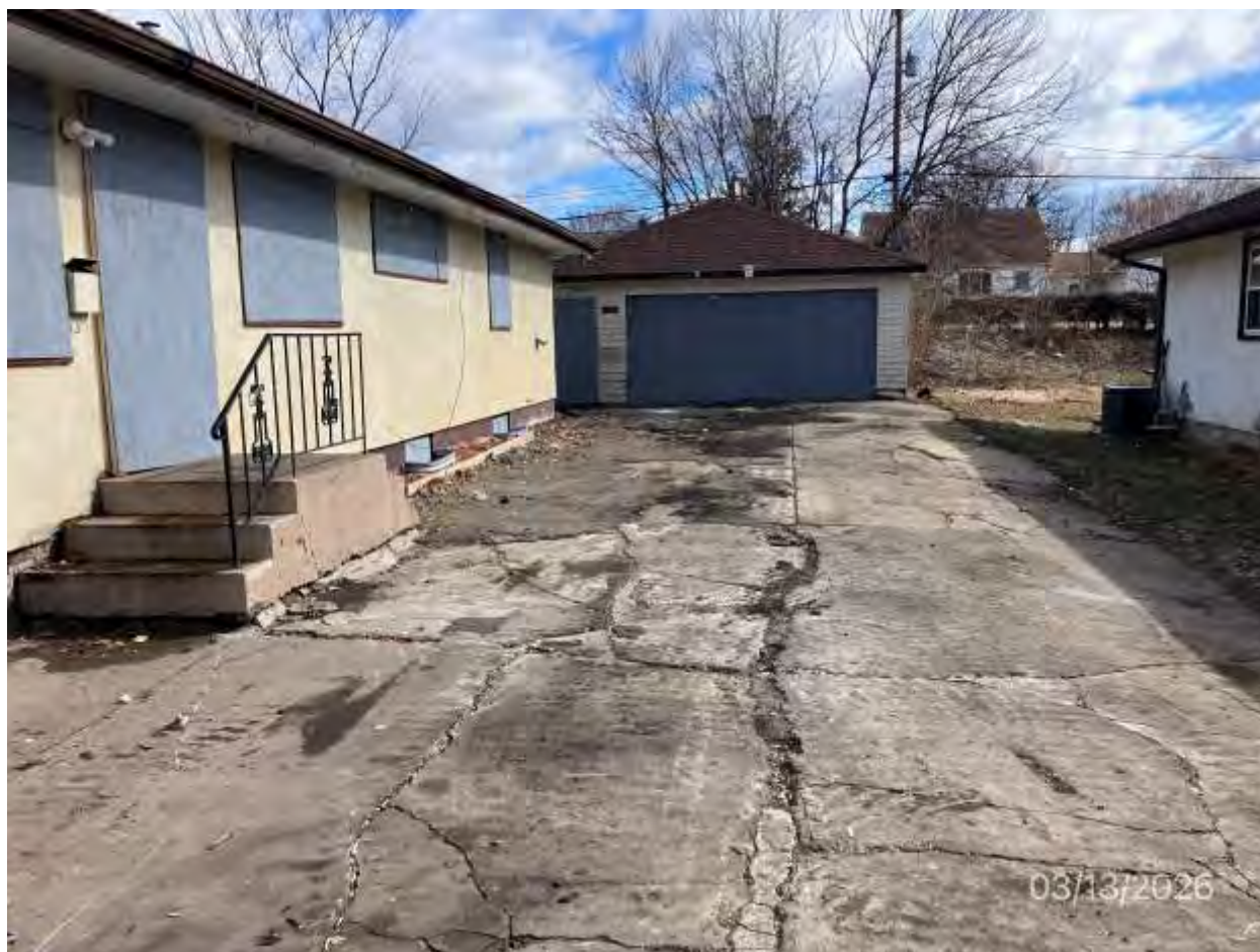
1164-1166 Cumberland St. Photos Before/After Clean Up 3-30-26
