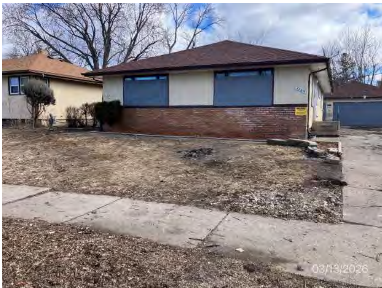
1164-1166 Cumberland St. Photos Before/After Clean Up 3-30-26
