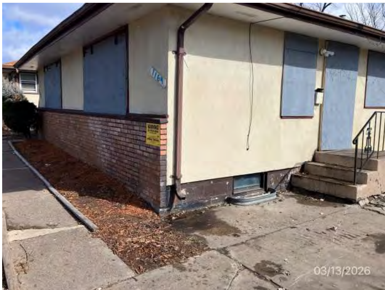
1164-1166 Cumberland St. Photos Before/After Clean Up 3-30-26
